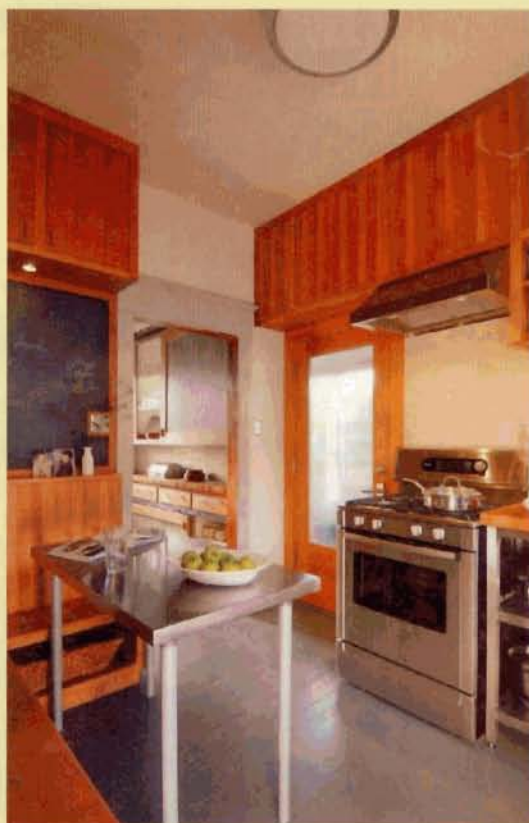
The kitchen's two adjoining rooms were reconfigured to improve work flow. Original fir flooring was refinished with low-VOC paint and AFM Polyureseal.
